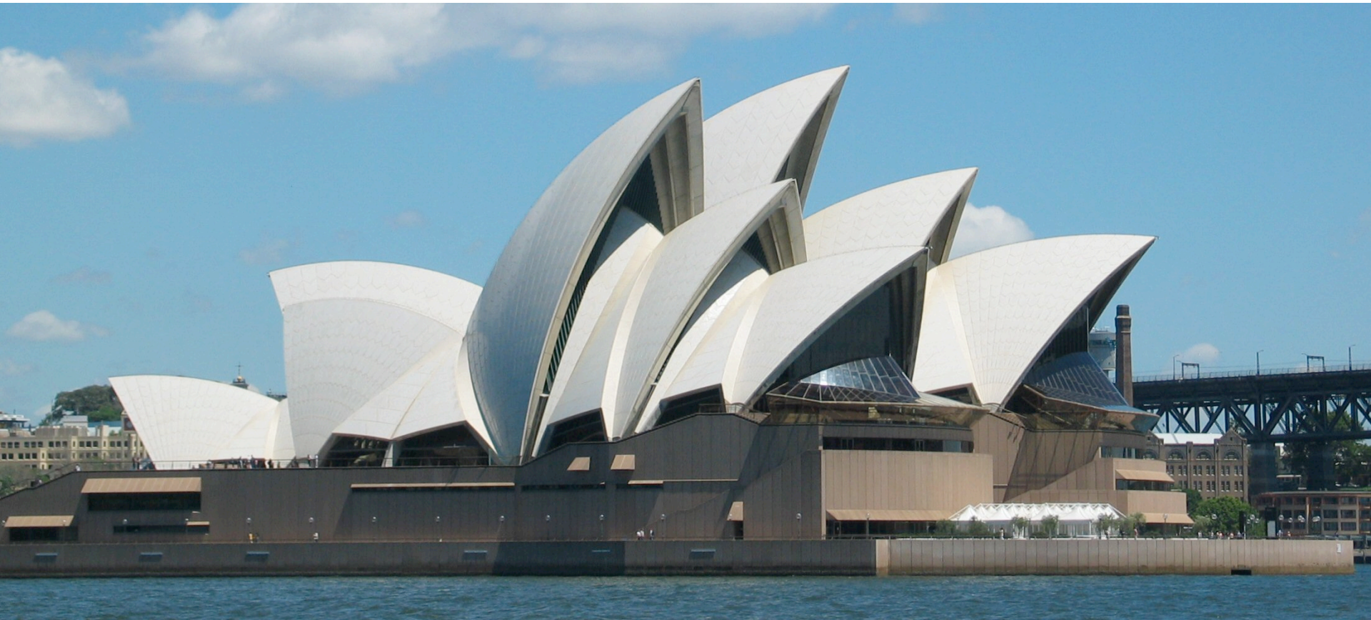
Sydney Opera House , shell architecture, by Danish architect Jorn Utzon, Sydney, Australia 1973
