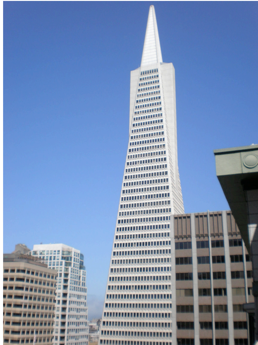
Transamerica Building, skeleton and skin architecture, San Francisco, California, USA 1972
