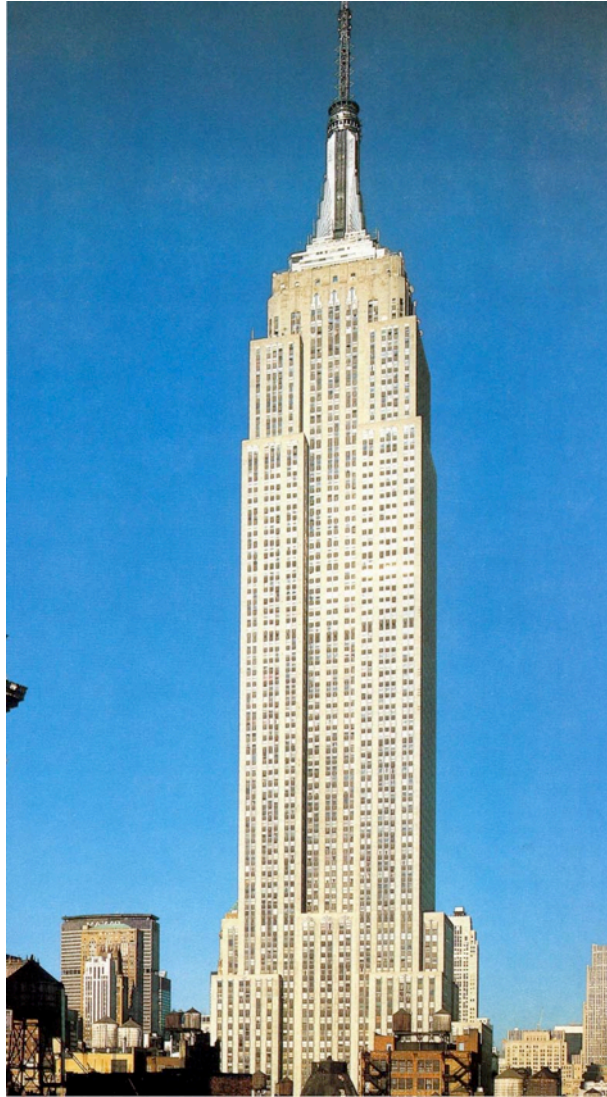
Empire State Building , skeleton and skin architecture, Art Deco style, New York City, New York, USA 1931 AD
