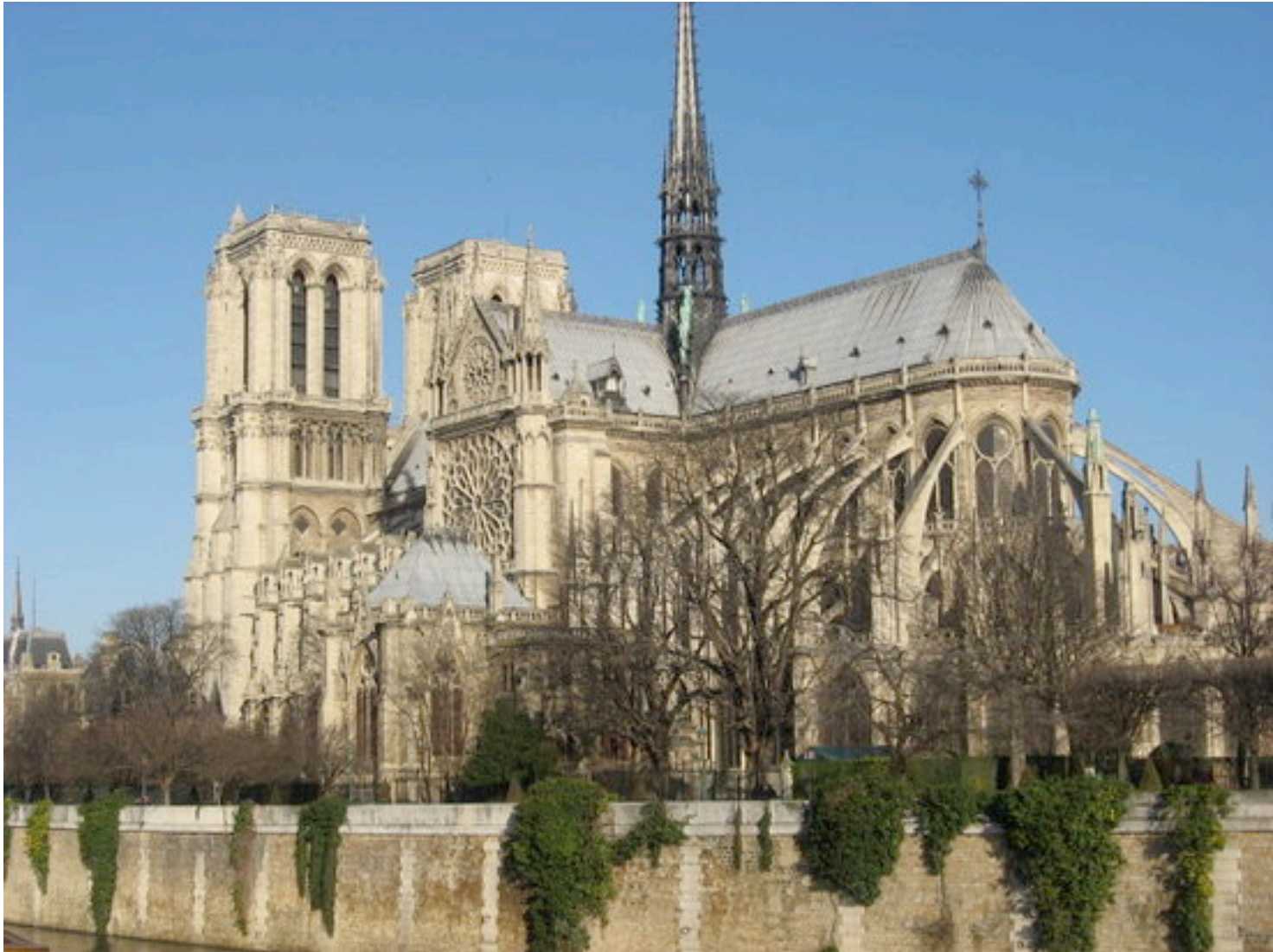
Notre Dame Cathedral, Paris, France completed 1260 AD
