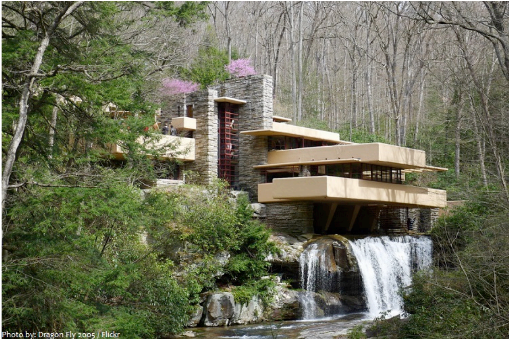
Falling Water home , by Frank Lloyd Wright, cantilever extensions, rural Pennsylvania, USA 1935
